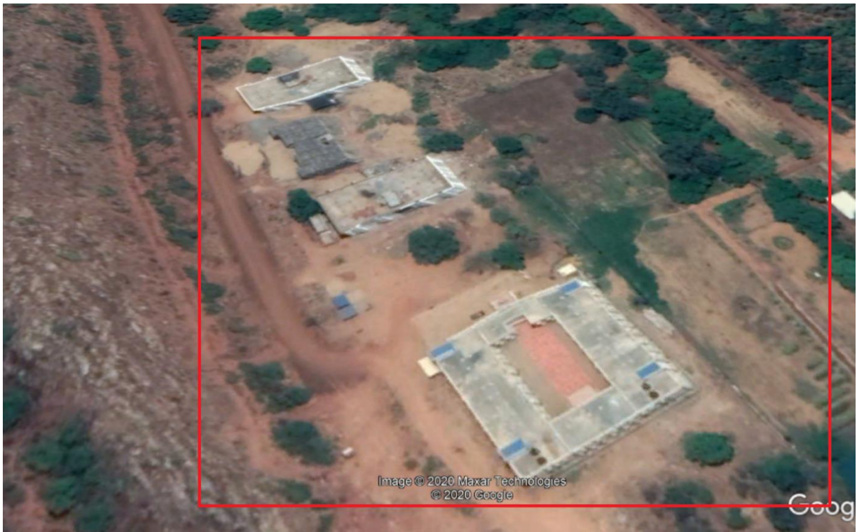
Figure 1 Srikalahasti Temple, Proposed Rooftop Location
